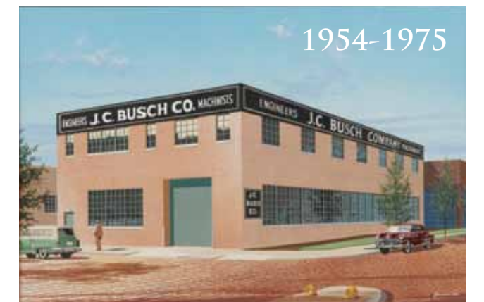
185 SOUTH BARCLAY STREET - HISTORIC 3RD WARD
